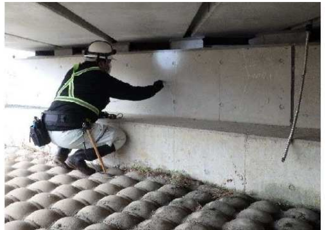
橋梁定期点検 (幸主橋)
